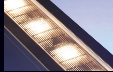
Micro louvre for glare control
