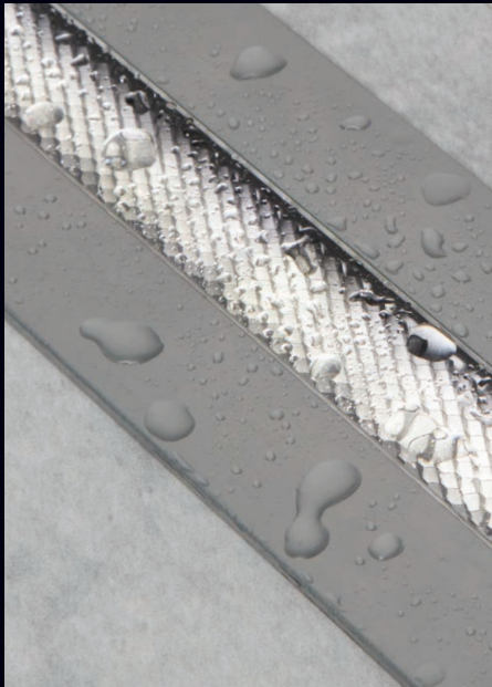
60 Honeycomb louvre for glare control
